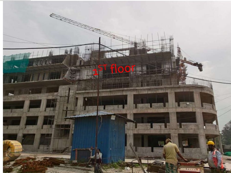
TOWER - B : 2 ND FLOOR TO 3 RD FLOOR SLAB ALUMINIUM SHUTTERING WIP
